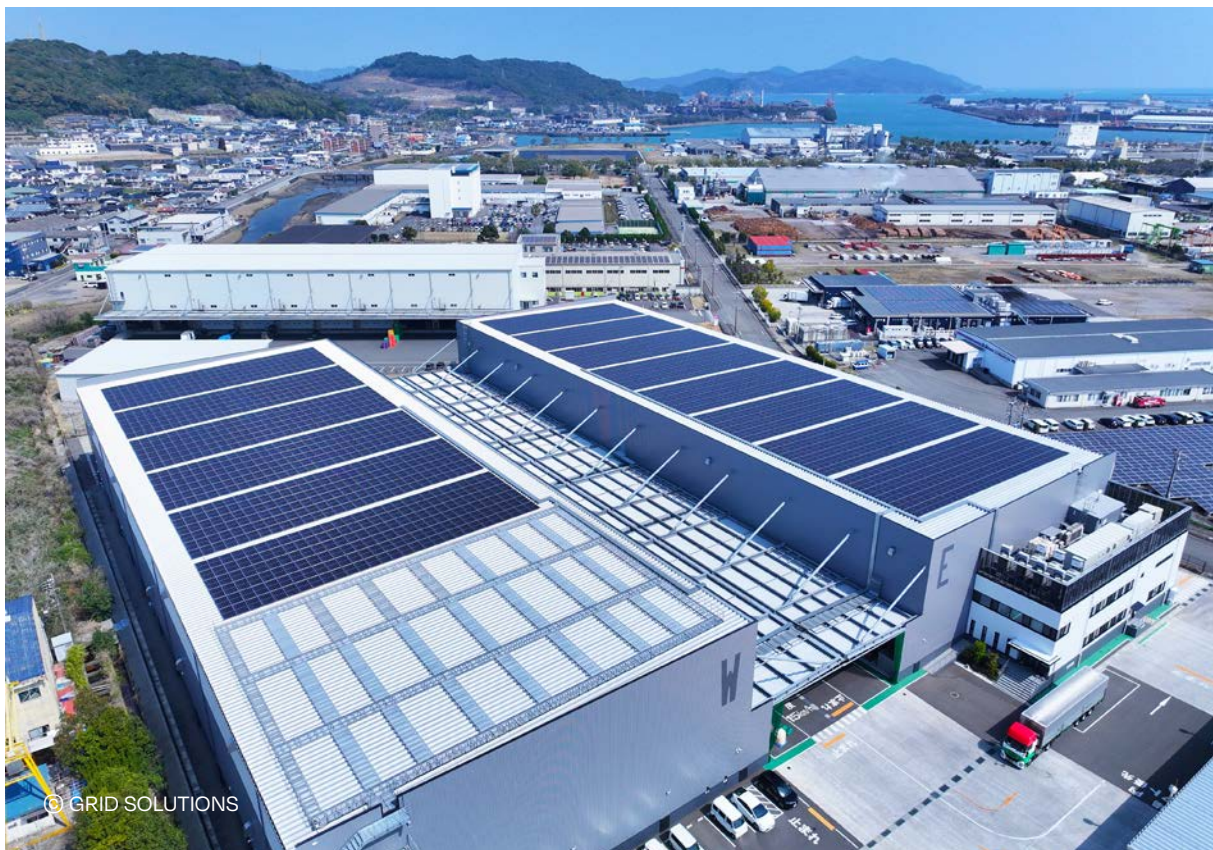
Rooftop solar PV, SENKO No.2 PD Center, on-site PPA model, Hakusan City, Japan
