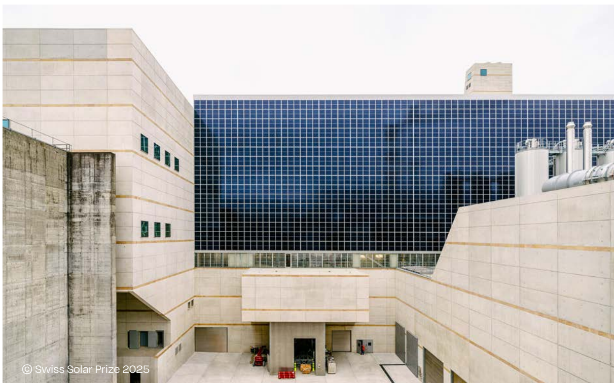
190 kW roof + 1178 kW façade solar PV, Kenova AG waste incineration plant, Zuchwil, Switzerland
