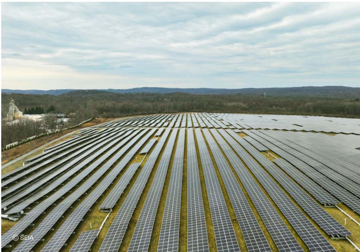
25.6 MW Mount Olive Solar Project, New Jersey, United States
