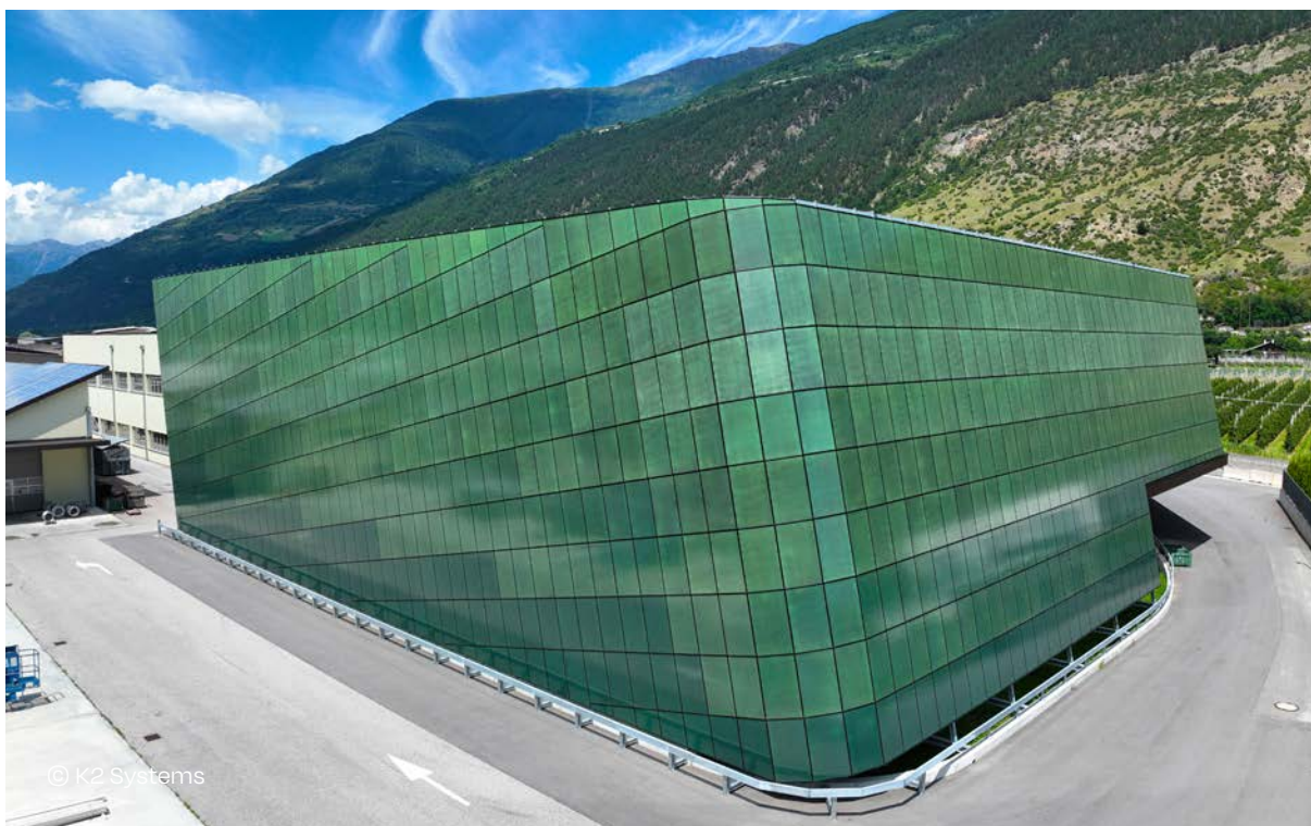
Façade PV system, Heerbrugg, Switzerland — 275 kW on a 25-metre-high façade
