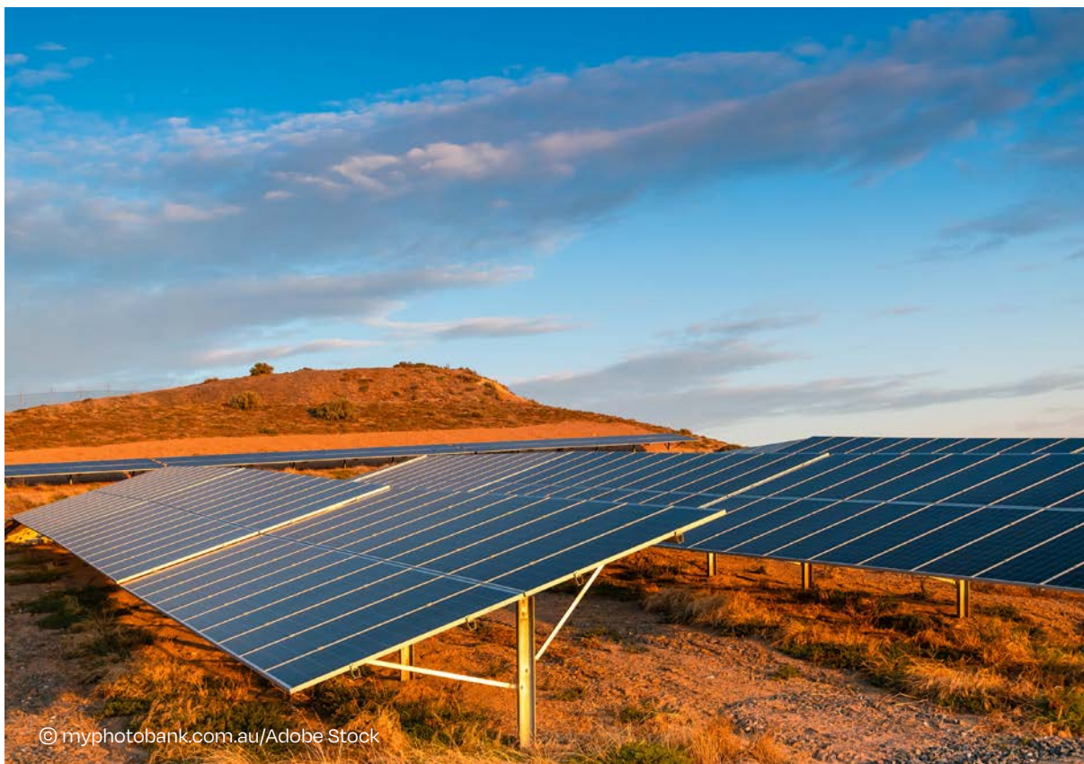
Suburban solar farm at sunset in Adelaide, South Australia
