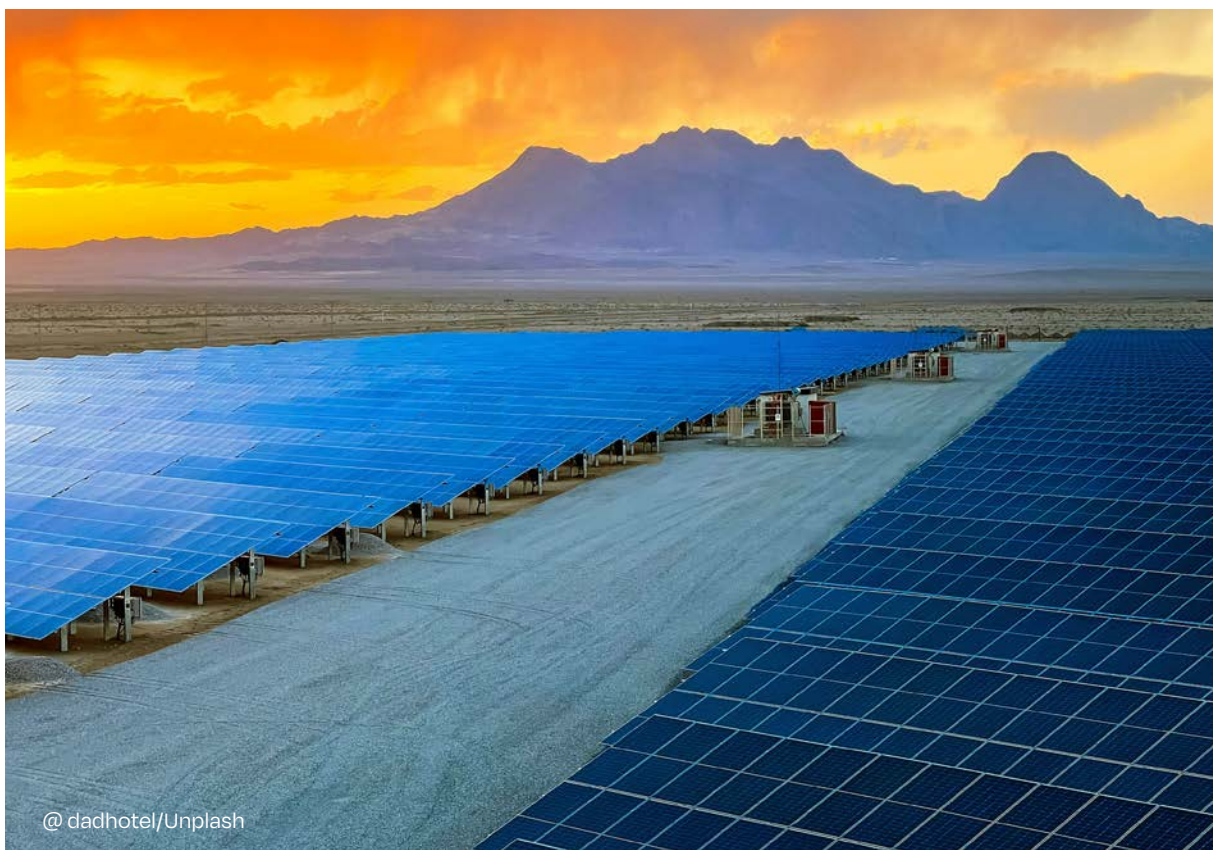
10MW solar power plant, Yazd Province, Iran
