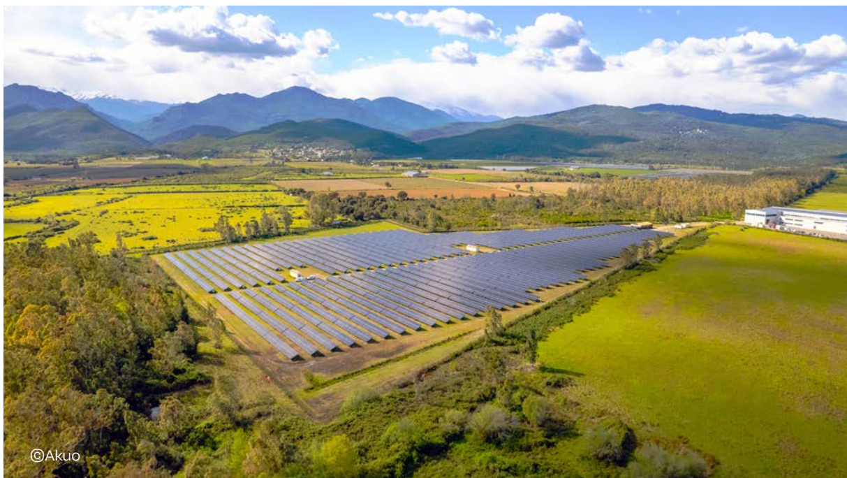
4.1 MWh / 4MW, Corsica, France
