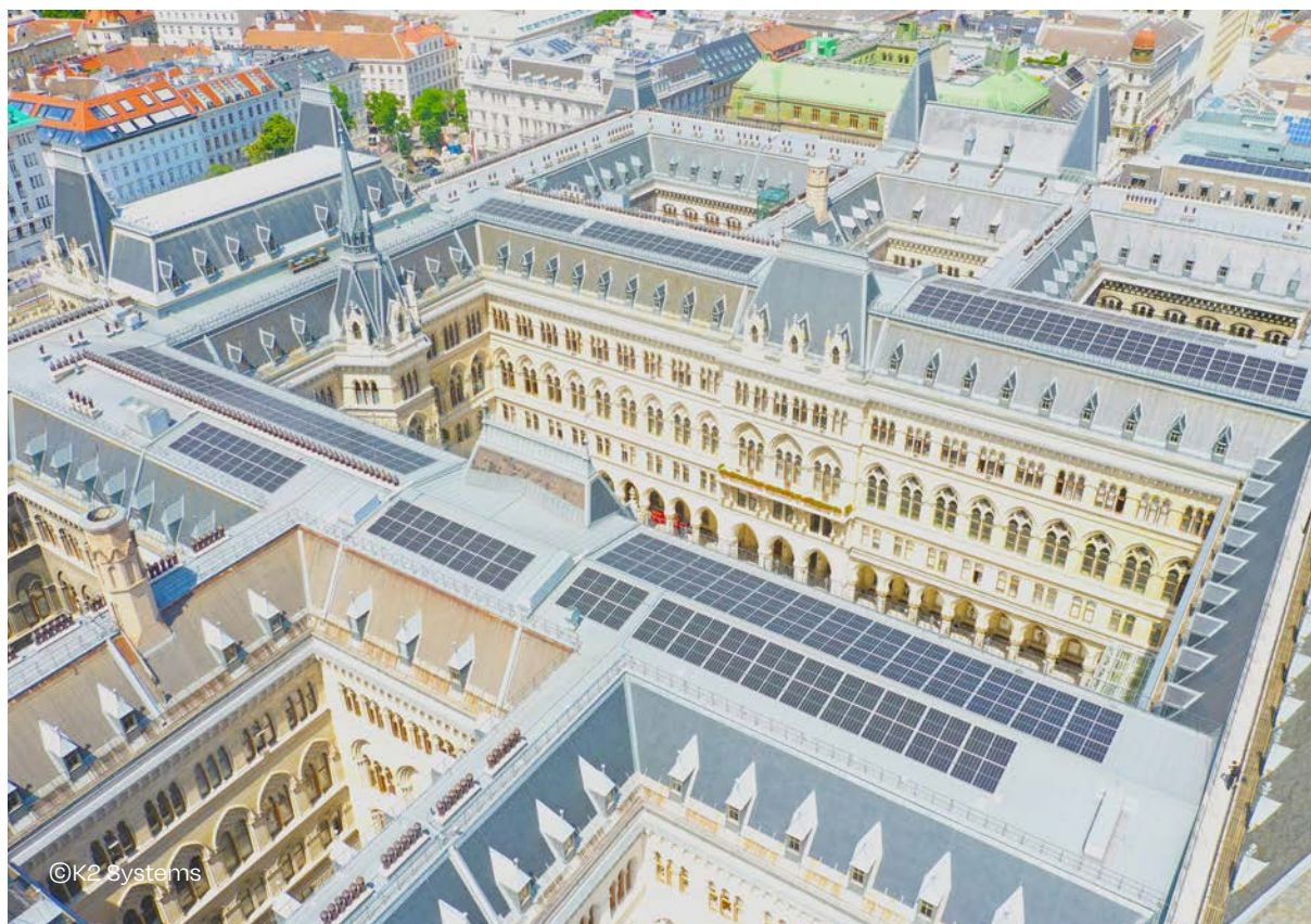
235 kWp on Vienna City Hall
