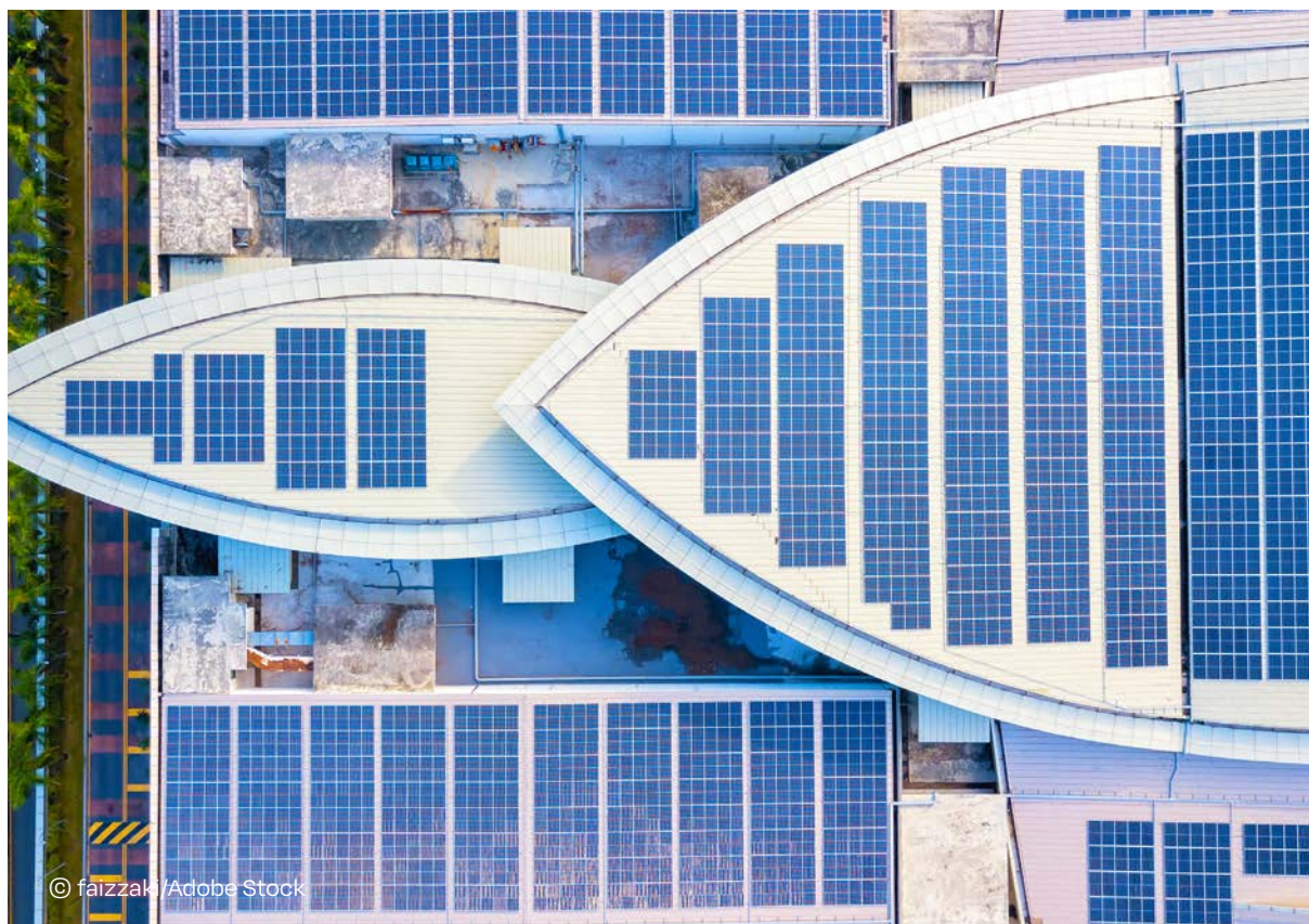
Solar panels on top of commercial building, Putrajaya, Malaysia
