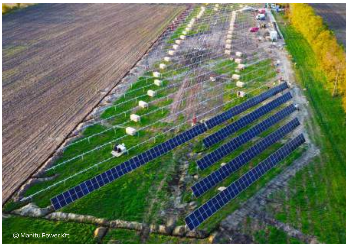
1 MW 1 axis tracker installed PV plant under construction in Komárom-Esztergom County, Hungary
