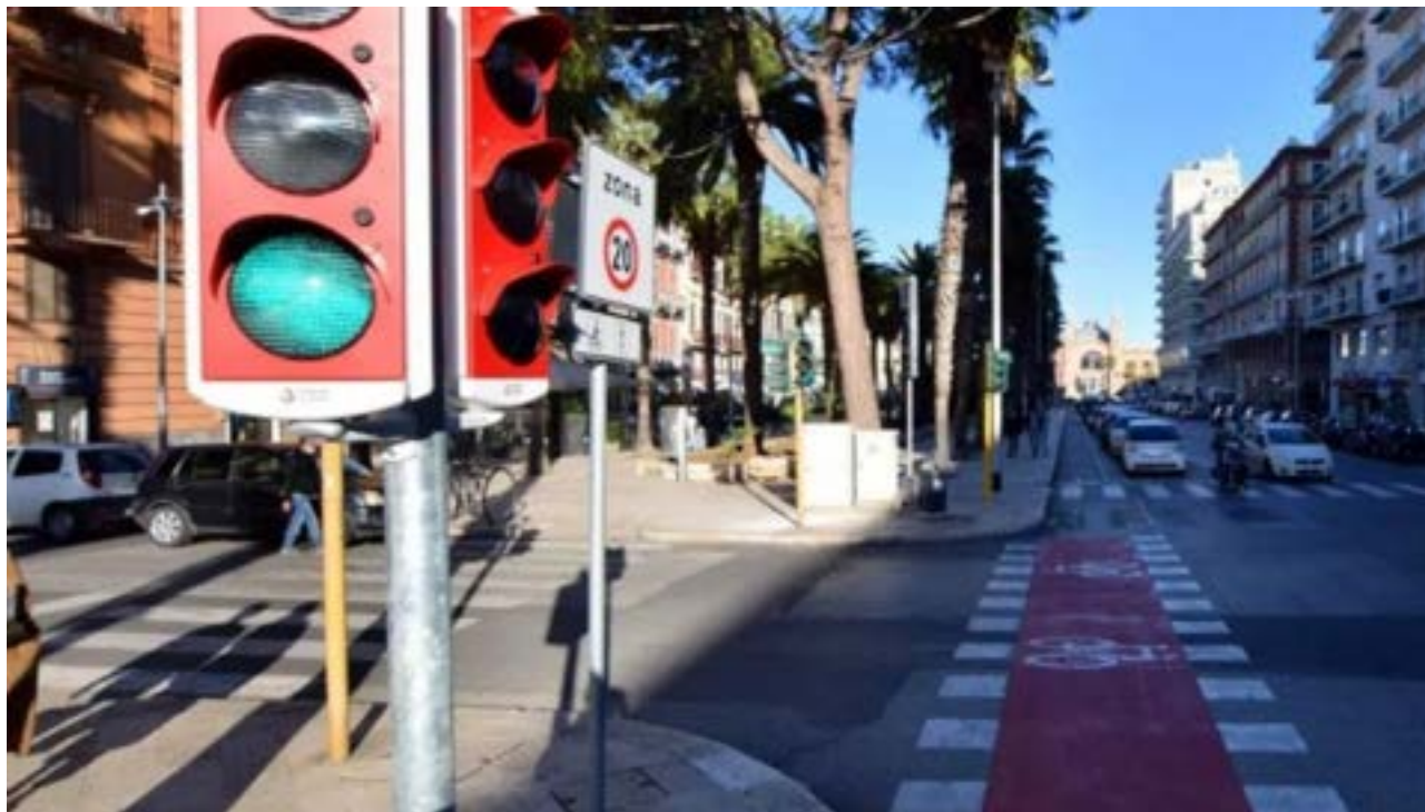
Figure 19 Installation of new traffic light systems
