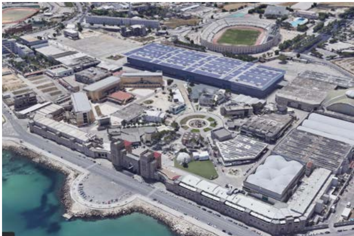
Figure 17 Views of the replication area 3
