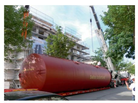
The core component of the building's heating system is a 72 m<sup>3</sup> steel tank, incorporated into the base build in October 2020. With a diameter of 2.3 m and a height of 17.8 m, it extends to all floors of the house. Photo: VolkMer ZichNer
