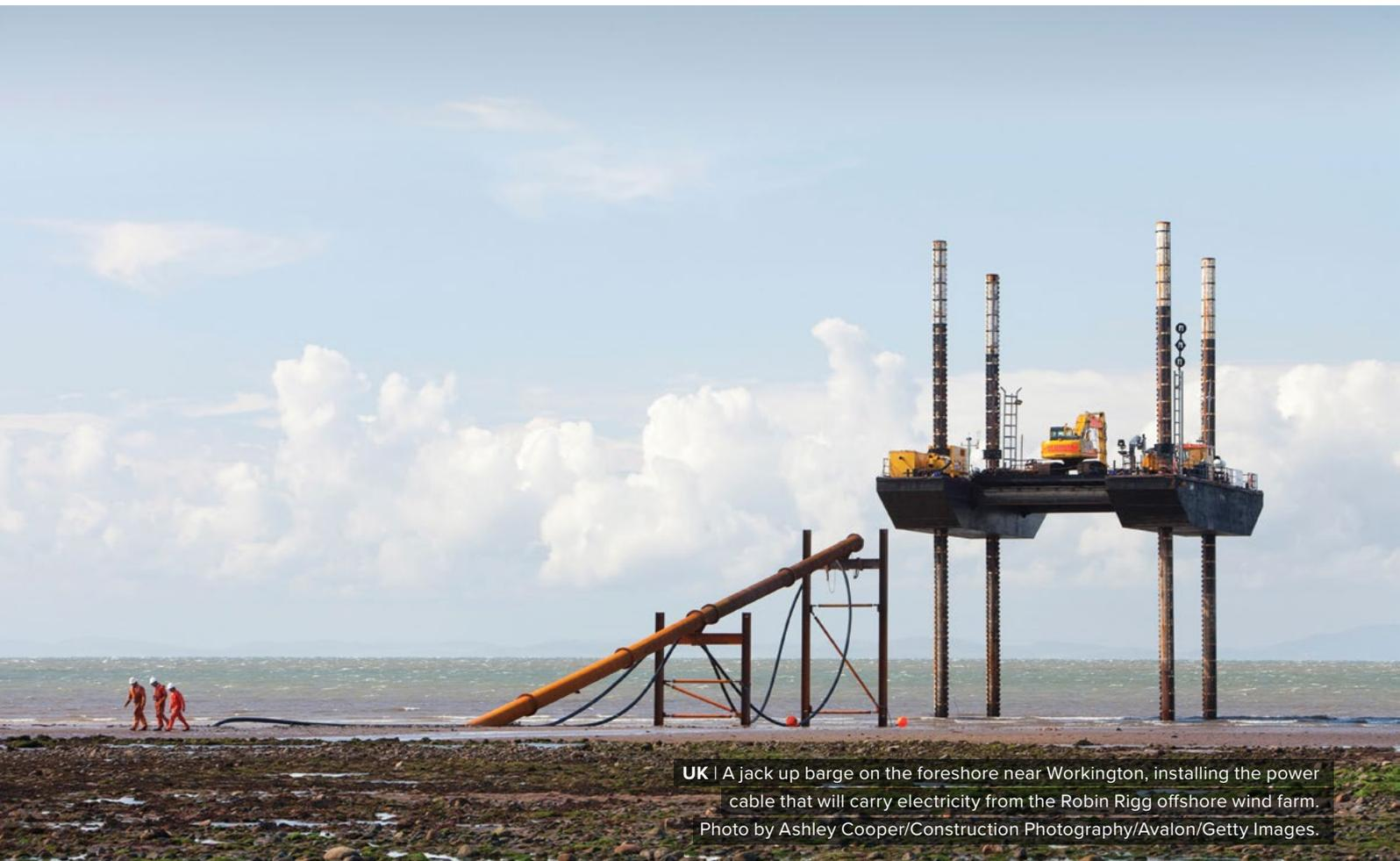
**UK** | A jack up barge on the foreshore near Workington, installing the power cable that will carry electricity from the Robin Rigg offshore wind farm. Photo by Ashley Cooper/Construction Photography/Avalon/Getty Images.
