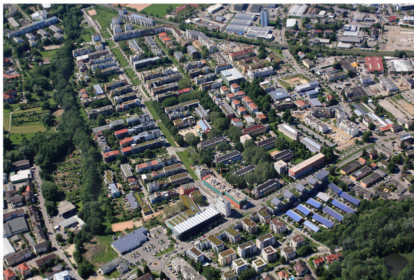
Fig. 5 Aerial view of Vauban neighbourhood in Freiburg, Germany. Copyright permission by Erich Meyer, Hasel|Stadt Freiburg (2012)
